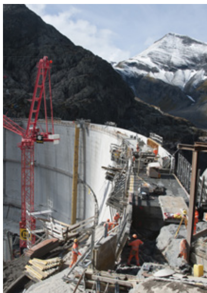
The 20-metre increase in the Vieux-Emosson dam to 76.5 metres doubles reservoir capacity. Vieux-Emosson forms part of the Nant de Drance pumped storage power station. This will offset volatile wind and solar power plant production from 2018, allowing consumption peaks to be met, such as for rail transportation. The power plant is set up for production capacity of 2.5 billion kWh of peak energy per year.
