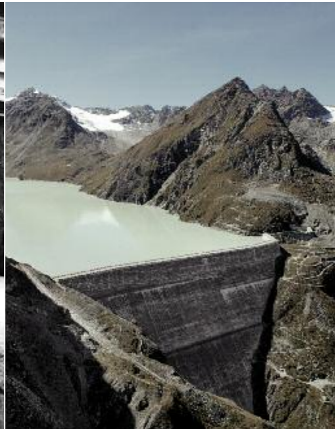
Grande Dixence dam
