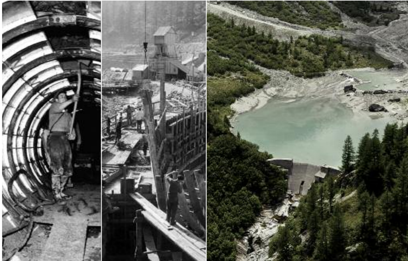
Concreting the Serra - Gondo inlet tunnel in 1951
