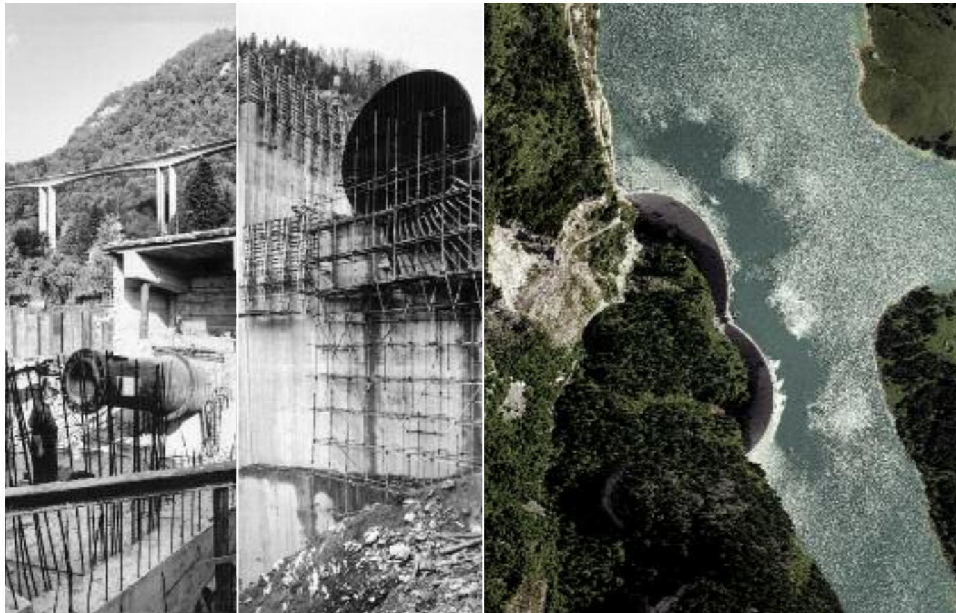
Veytaux: construction of the Léman hollow-jet valve in the nineteen seventies
